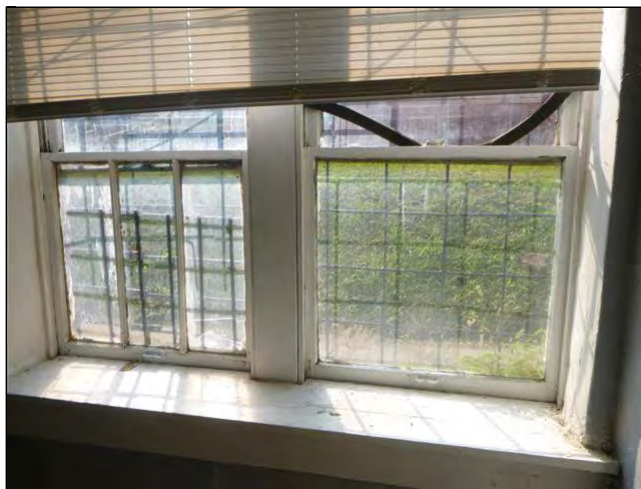
11.0 30 Unit 3 - Lower Level
