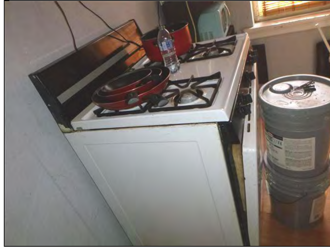
10.0 2 Paint buckets hold the door closed while cooking. Better than cans of Paint Thinner, but...
