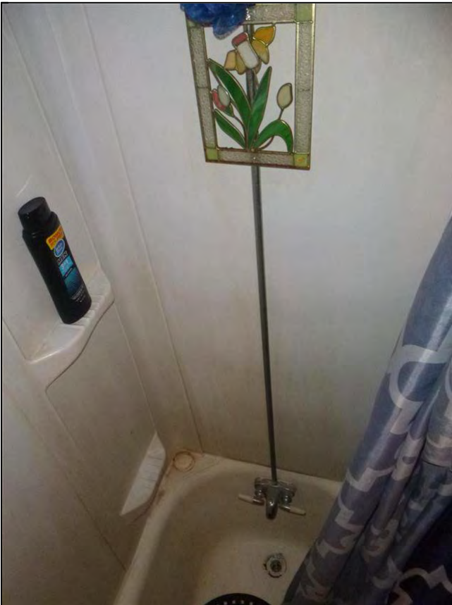
11.0 21 Unit 1 lower level
