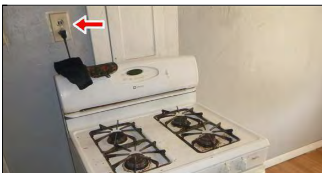
6.5.1 Example of one of dozens needed
