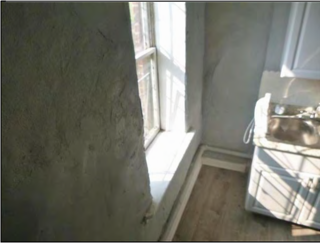
11.0 25 Unit 3 - Lower Level
