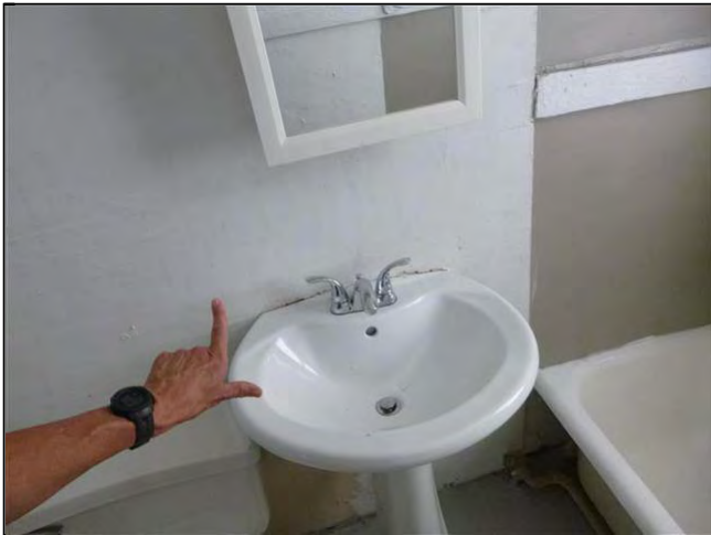
7.1 7 (6) Leaking devices noted at #3 Sprayer in Kitchen, which also has a slow-draining, debris-clogged tub
