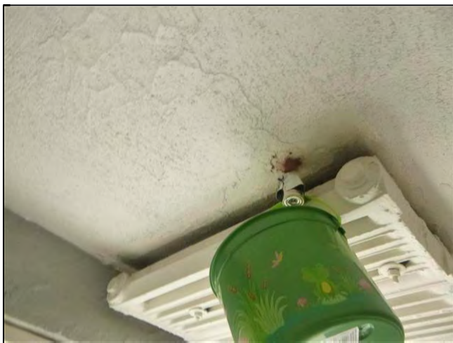
11.0 29 Unit 3 - Lower Level
